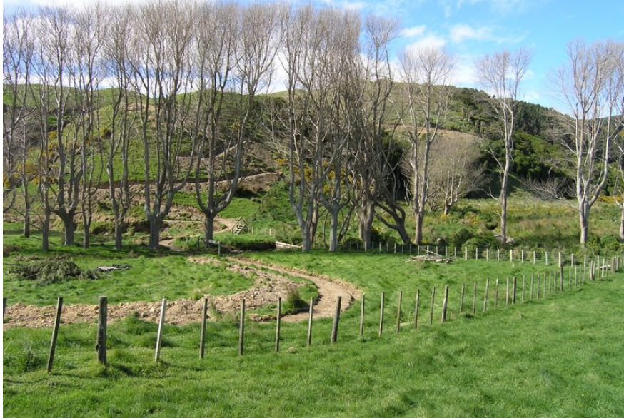
New track under construction
