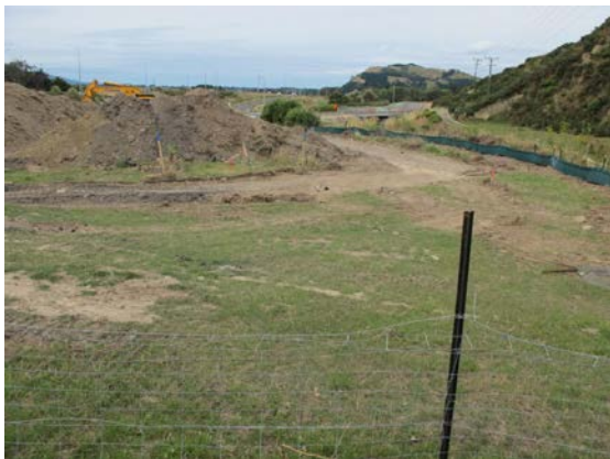
Waterfall Rd earthworks
