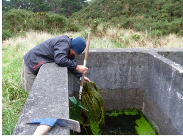
Liffet clearing weed out of water intake settlement chamber
