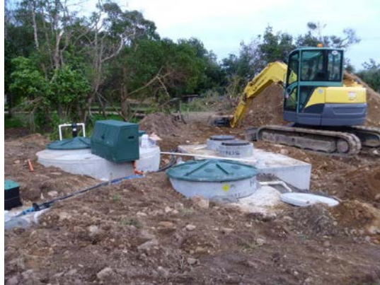
Work on new sewage system for entrance toilets
