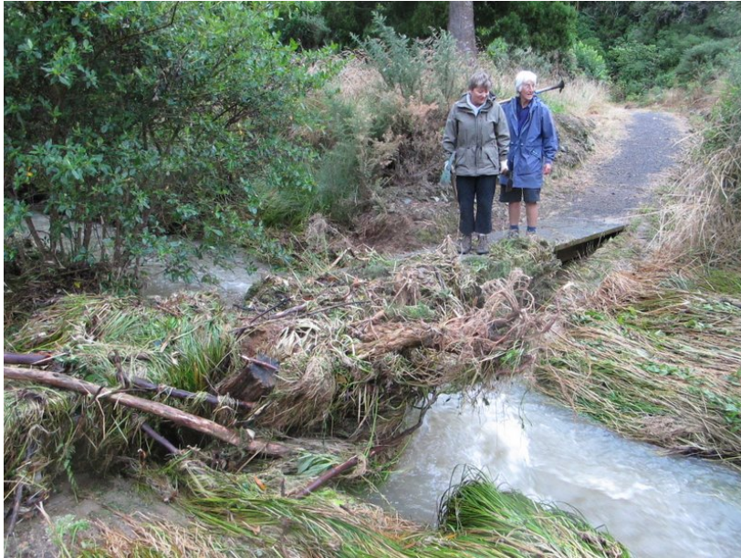
The foot bridge at the end of the bush walk
