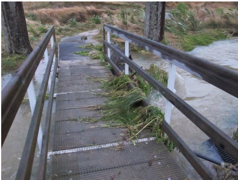
The foot bridge in the entrance picnic area.
