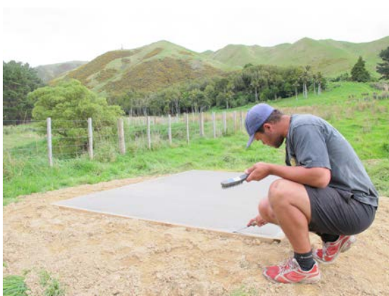
Sascha laid the concrete pads
