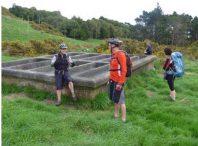
Water intake to be fenced for child safety
