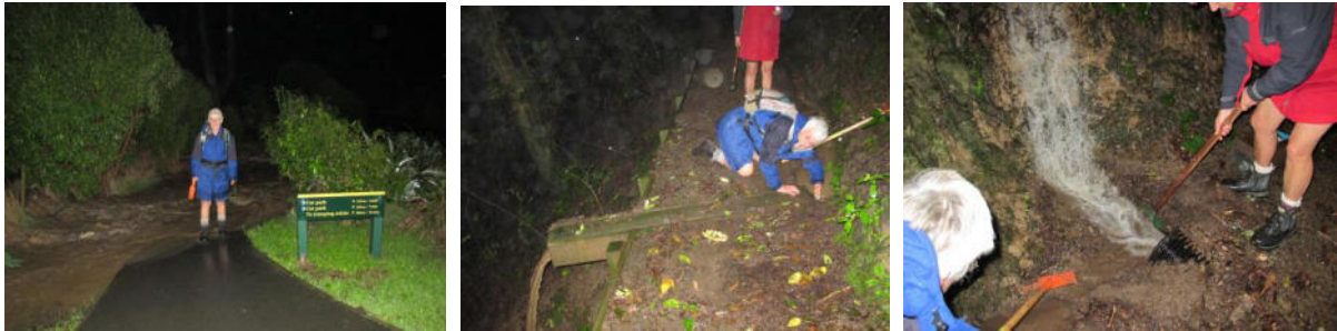
6.30am May 14 th . Morning Maintenance Gang: clearing culverts
