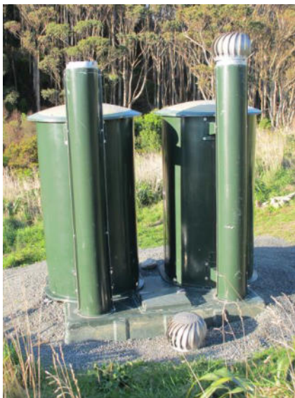
The "Kremlin" has lost its top, a piece inside is broken. The fans dry the contents of the tank and stop it smelling.
