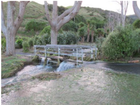
Water still flowing over the bridge
