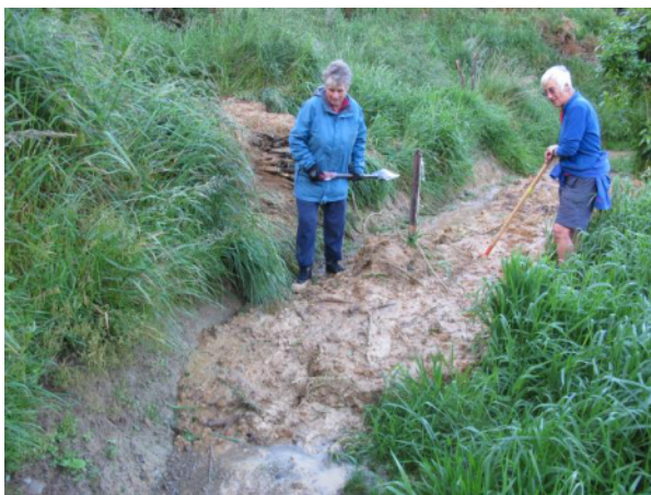
Slip across Upper Dell Track
