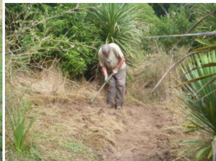
Dave chipping away at the track
