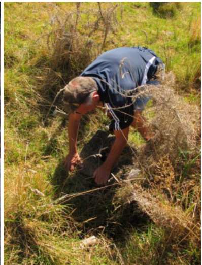
Gavin investigating water supply valves
