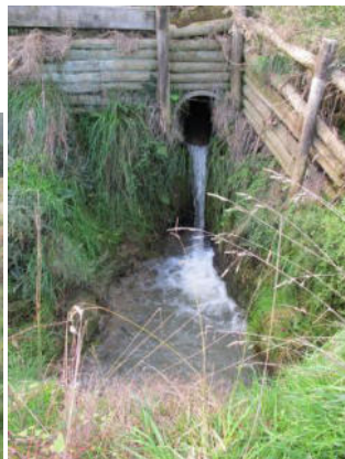
Culvert carrying reservoir overflow
