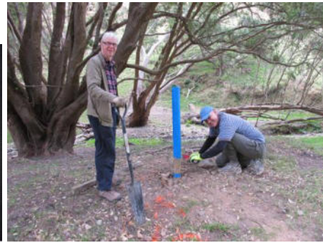
Peter & Bernard putting up posts on Ramaroa
