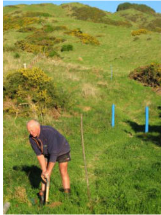
John putting in post for sign
