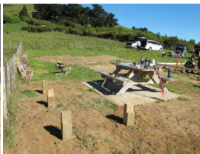
Piles ready for bench seat
