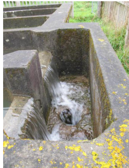
Overflow takes excess back to the stream
