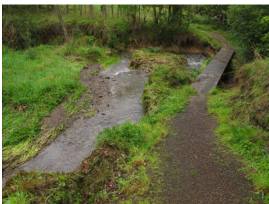
Heavy rain March 22 nd & 24 th - damage at end of the Forest Loop Walk by washing down the track and bank erosion
