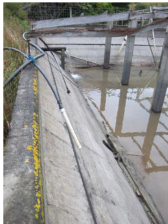
Outlet pipe exposed where water had drained away Water inflow Reservoir filling up again after repairs
