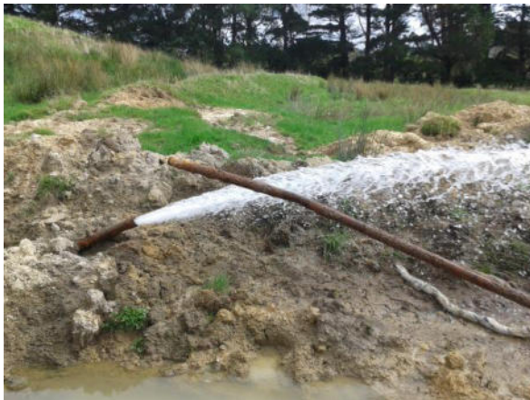
Burst pipe geyser, April 2017
