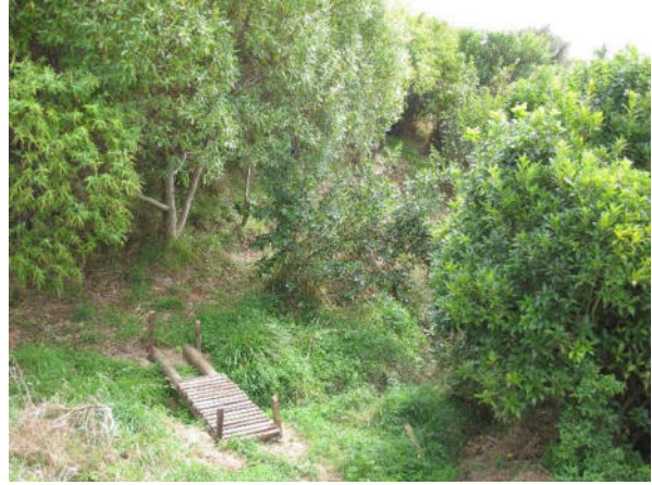
Theo's work in progress, Upper Ti Kouka Loop, recycling fences
