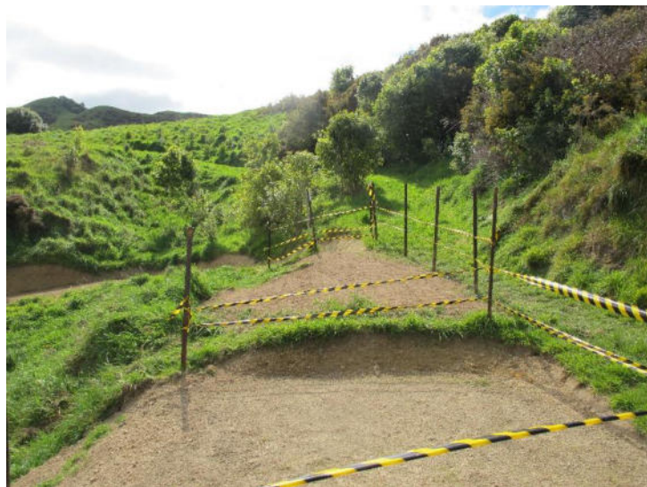
Final touches and grass seeding of Upper Dell Loop Track
