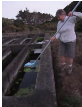
Liffet clearing intake
