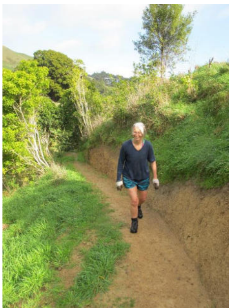
Sarah on the new track (waiting for topsoil & grass)
