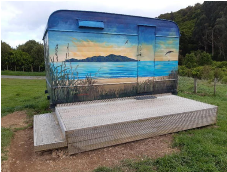
The finished job, deck is level again.
