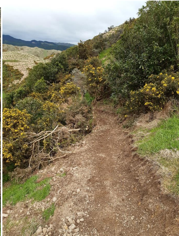
Part of the new route
