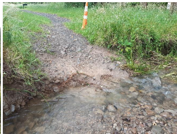
Erosion of main track by Gums (Bruce repaired)
