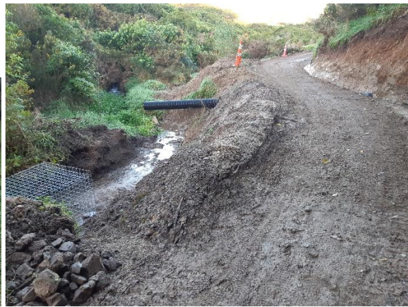
Track repaired, pipe & 1 st Gabion placed
